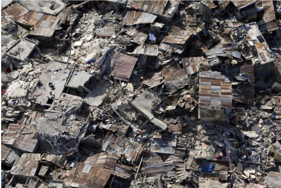
Picture - 2: Haitian-Truth.org (2010) Picture showing the massive destruction of an urban area in Léogâne.
