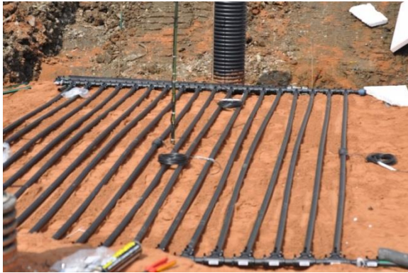
Ground temperature sensors Figure 2: (L) Installation of ground heat exchanger and (R) Infiltration trench and drainage pipe.
