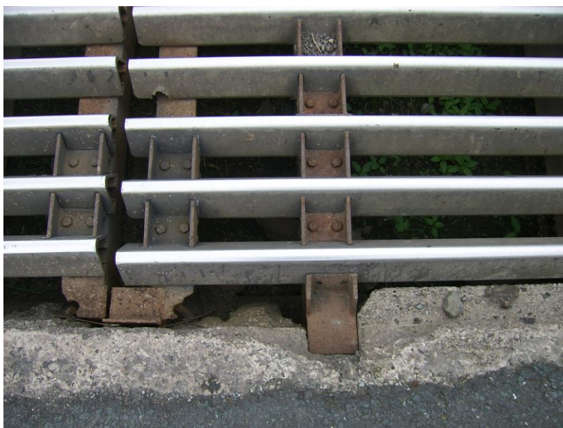
Figure 8: Damage to concrete support frame at Sedbergh B site
