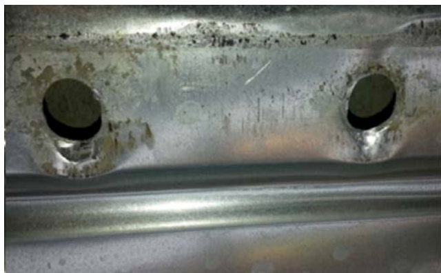
Fig. 6. Elongation of holes in the metal deck
