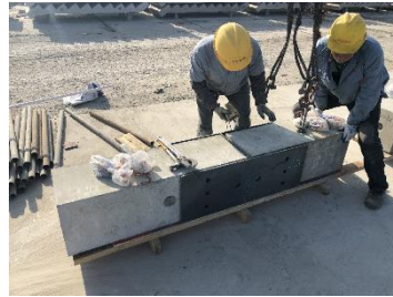
(e) Precast column assembly
