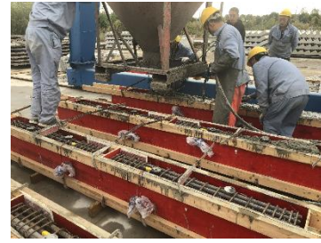
(c) Concrete pouring
