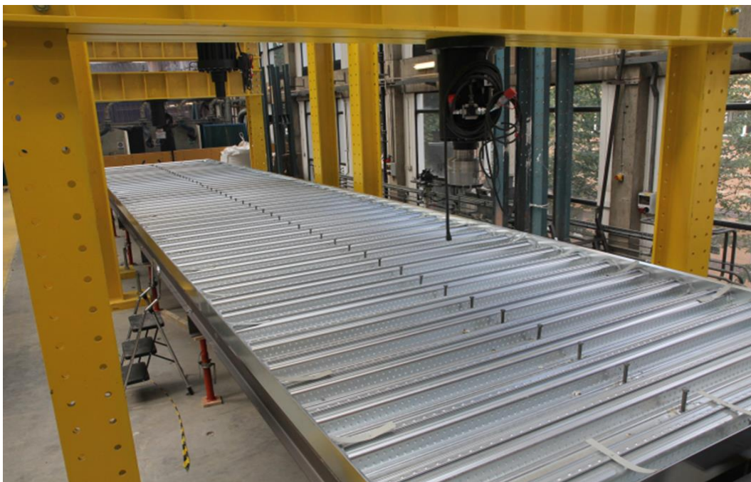
(b) after installation of profile decking and shear studs
