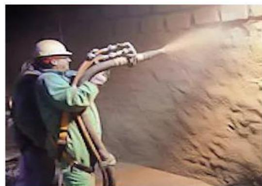
(d) Rehabilitation of pipelines and tunnels in place by shotcrete added with ConShield
